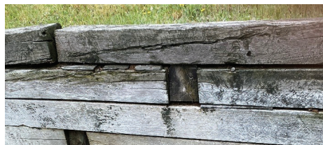
Treated wood retaining wall
