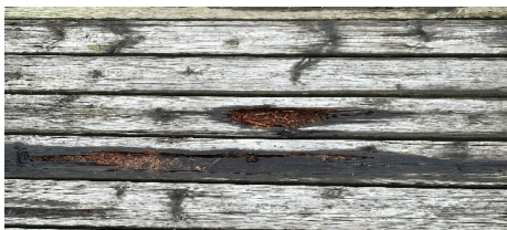
Treated wood walkway
